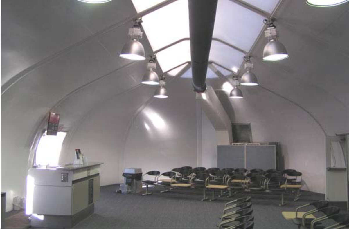
Example of Fabric Structure Building
