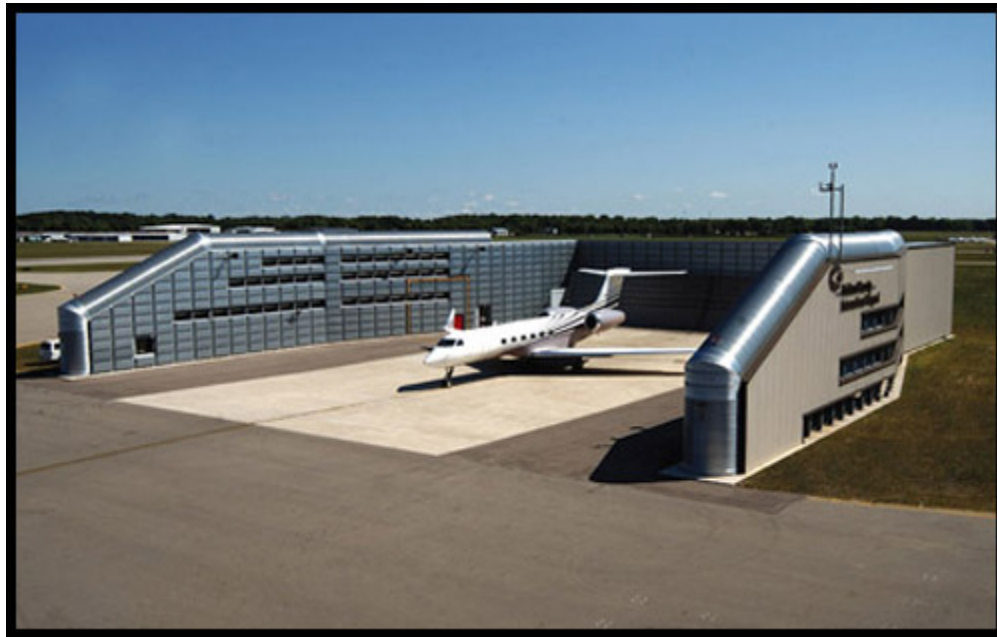
Figure 2 — Example of Ground Run-up Enclosure
