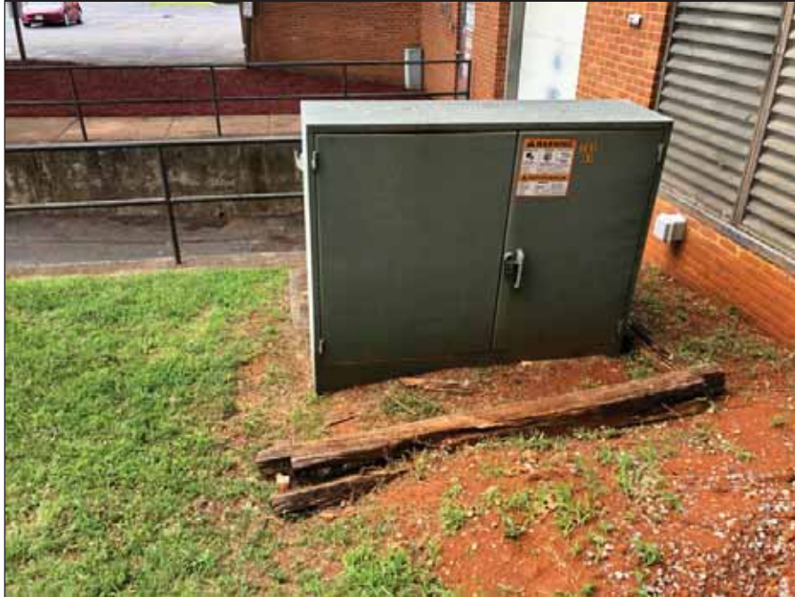
17 - Pad mounted transformer
