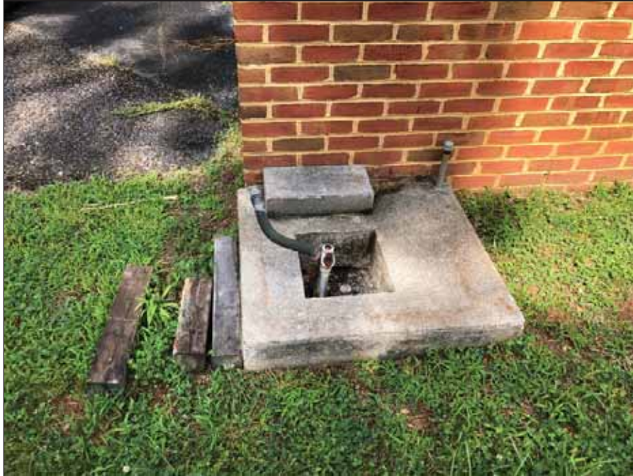
13 - Location of the pump for the 10,000 gallon UST on the north side of the hangar
