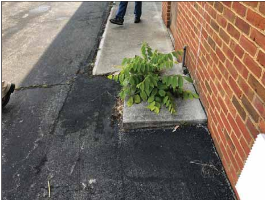
12 - Location of the former pump for the 10,000 gallon UST along the southside of the hangar
