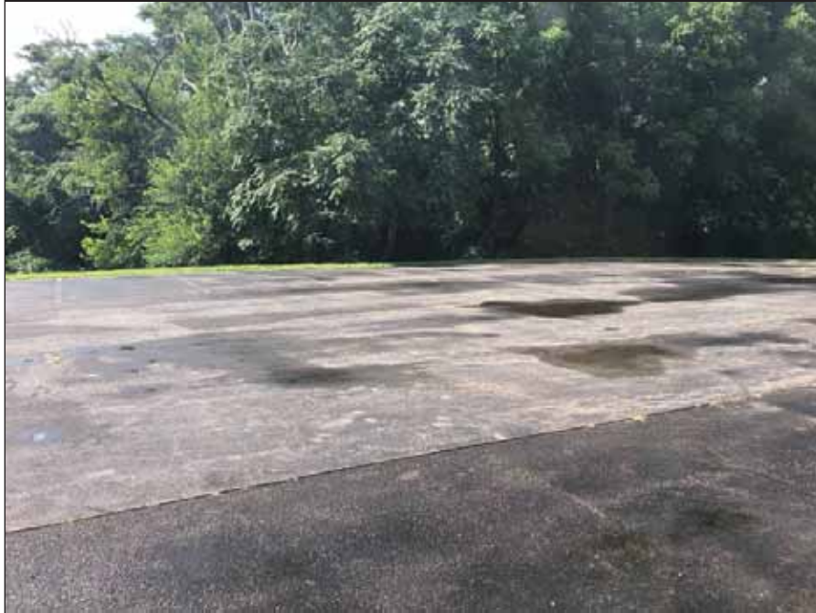
21 - Parking lot on the north side of the hangar
