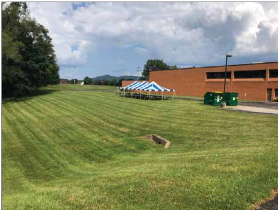
14 - Stormwater detention pond
