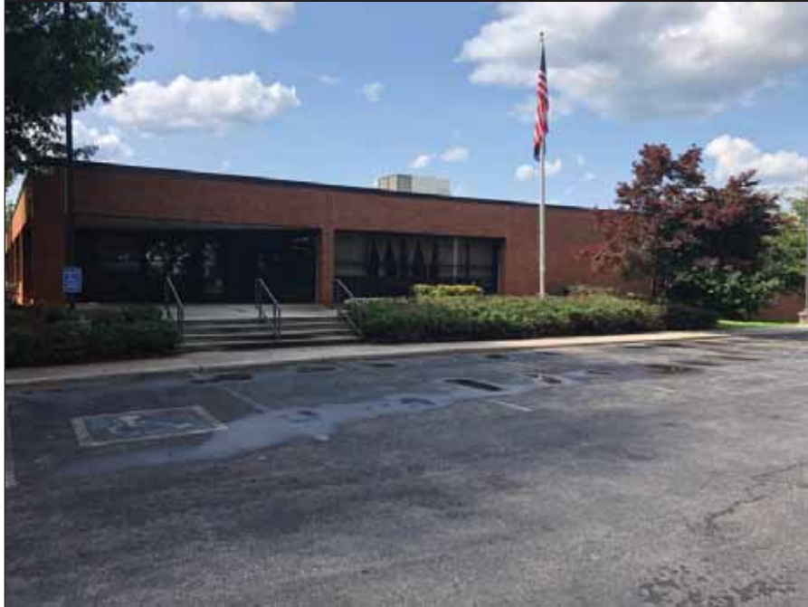
1 - Front of the manufacturing/office building
