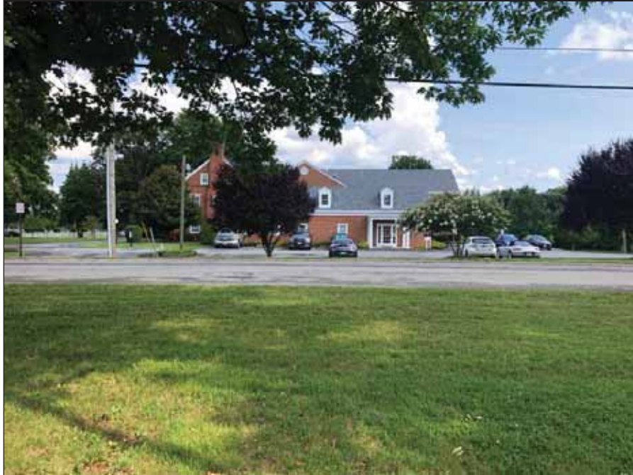
19 - Adjoining property to the south
