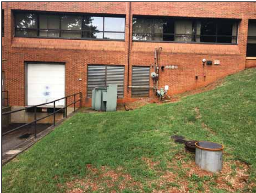
18 - The 4,000 gallon UST
