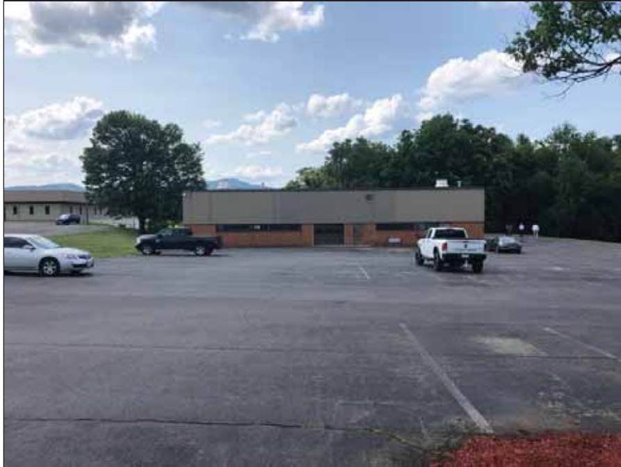
11 - The hangar building
